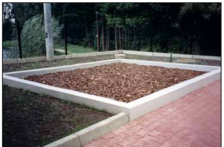
Biological Filtration Unit
