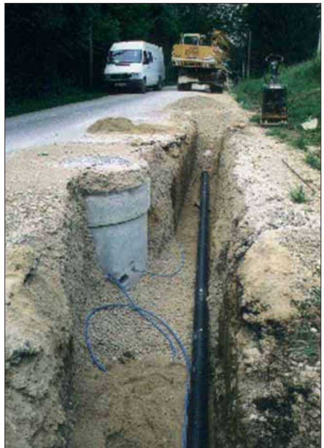
Laying of valve monitoring cable within sewer trench
