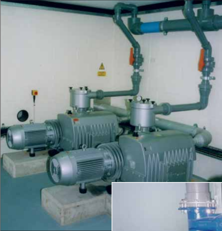
Rotary vane, single stage oil-sealed vacuum pumps
